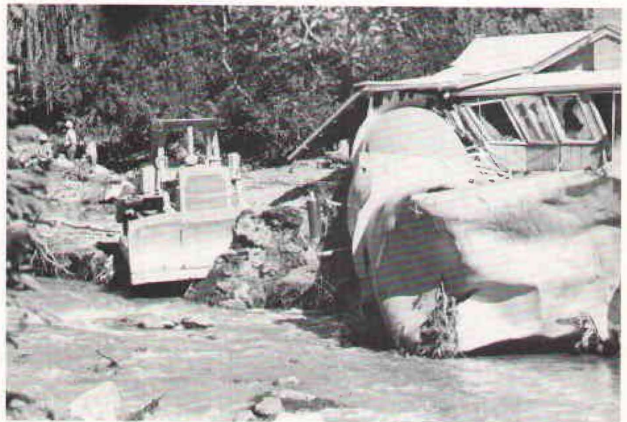
A siphon tube, nine feet in diameter, caught the full force of the huge wall of water and collapsed, slamming into this house. The scene is near the steep-walled area of the canyon known as the Narrows, a few miles west of Loveland.
