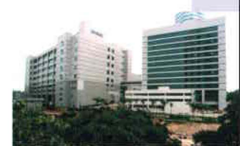
These HP Singapore buildings were completed in 1997.
