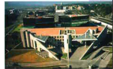
The Mexico City facility was built in two phases. The right side was completed in 1995 and the left side in 1997.
