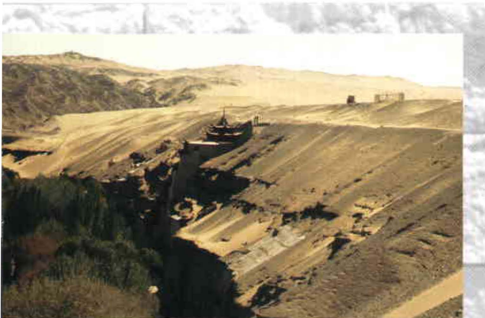
The Getty Conservation Institute and the State Bureau of Cultural Relics are preserving Mogao Grottoes—an ancient Buddhist site along the Silk Road in northern China. Buddhist monks cut hundreds of rock temples into the sandstone face near Dunhuang City from A.D. 366 to about 1300.
