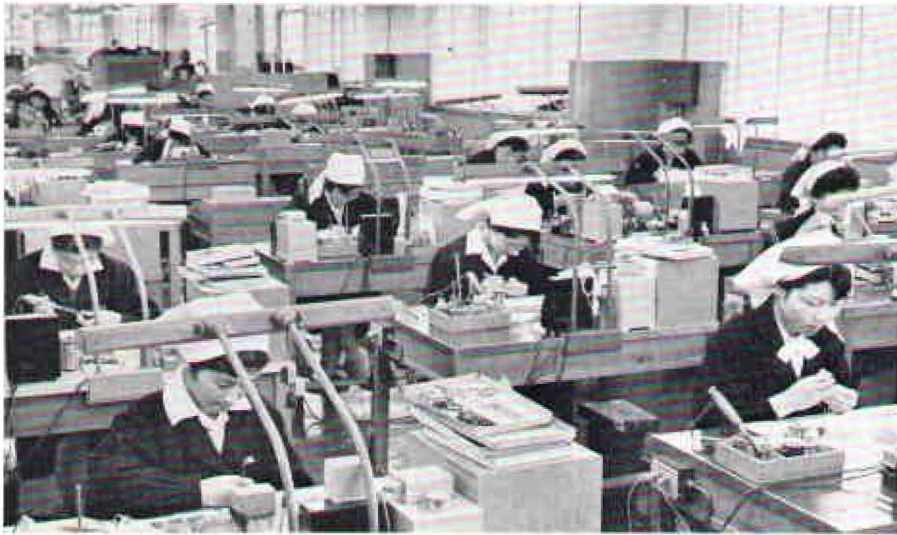
Production areas, such as electrical indicating instrument assembly line, are remarkably clean and orderly.
